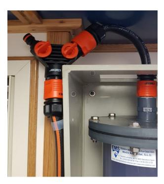
• Close white drain. Be sure to leave output handle open and input tank closed. Be sure to leave "Y" drain tank open.
