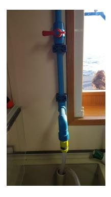
• Open "Y\_tank" pass above Thermosal tank to allow water volume to get in.
