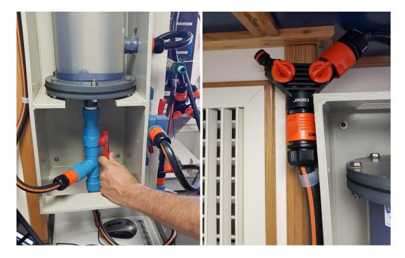
Connect fresh water hose to tank input.
